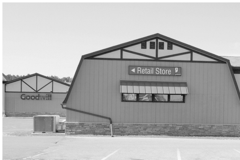
The 6,000 square foot Goodwill Retail and Donation Center in Gaylord is located at 1361 Pineview Drive. Photo by Jim Akans
